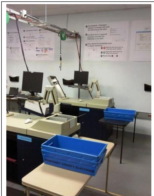
Figure 7 – Open Catwalks Give A Clear View of Cables
